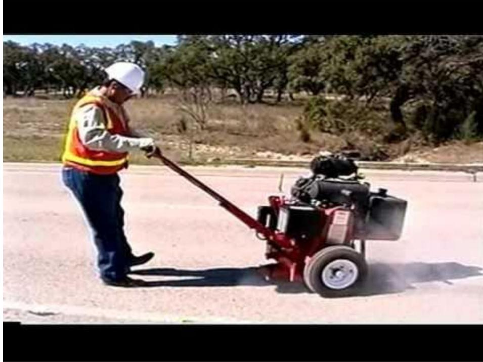
Crack Sealing Asphalt Pavement Video (part 2):
